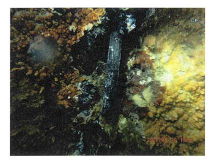
Severe condition of Pile 23B with exposed reinforcing
