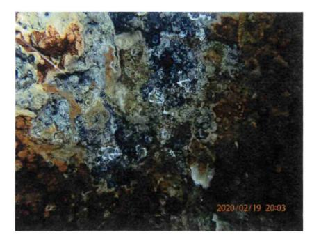
Erosion of pile chamfer at Pile 18B – Pile rated Major
