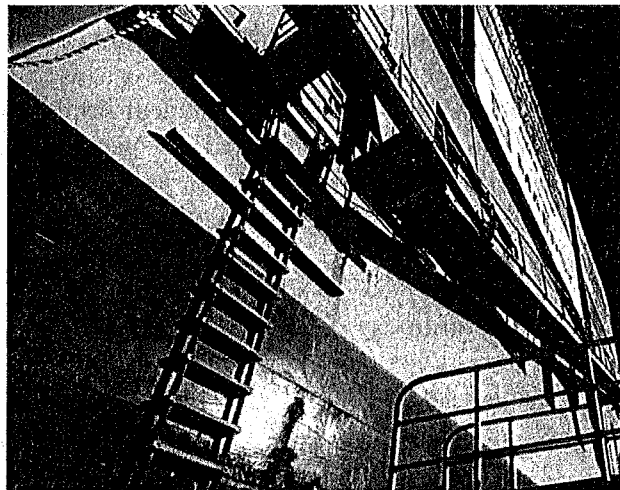
Example of trapdoor arrangement with ladder hanging from bottom of platform
