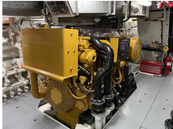
Starboard main engine
