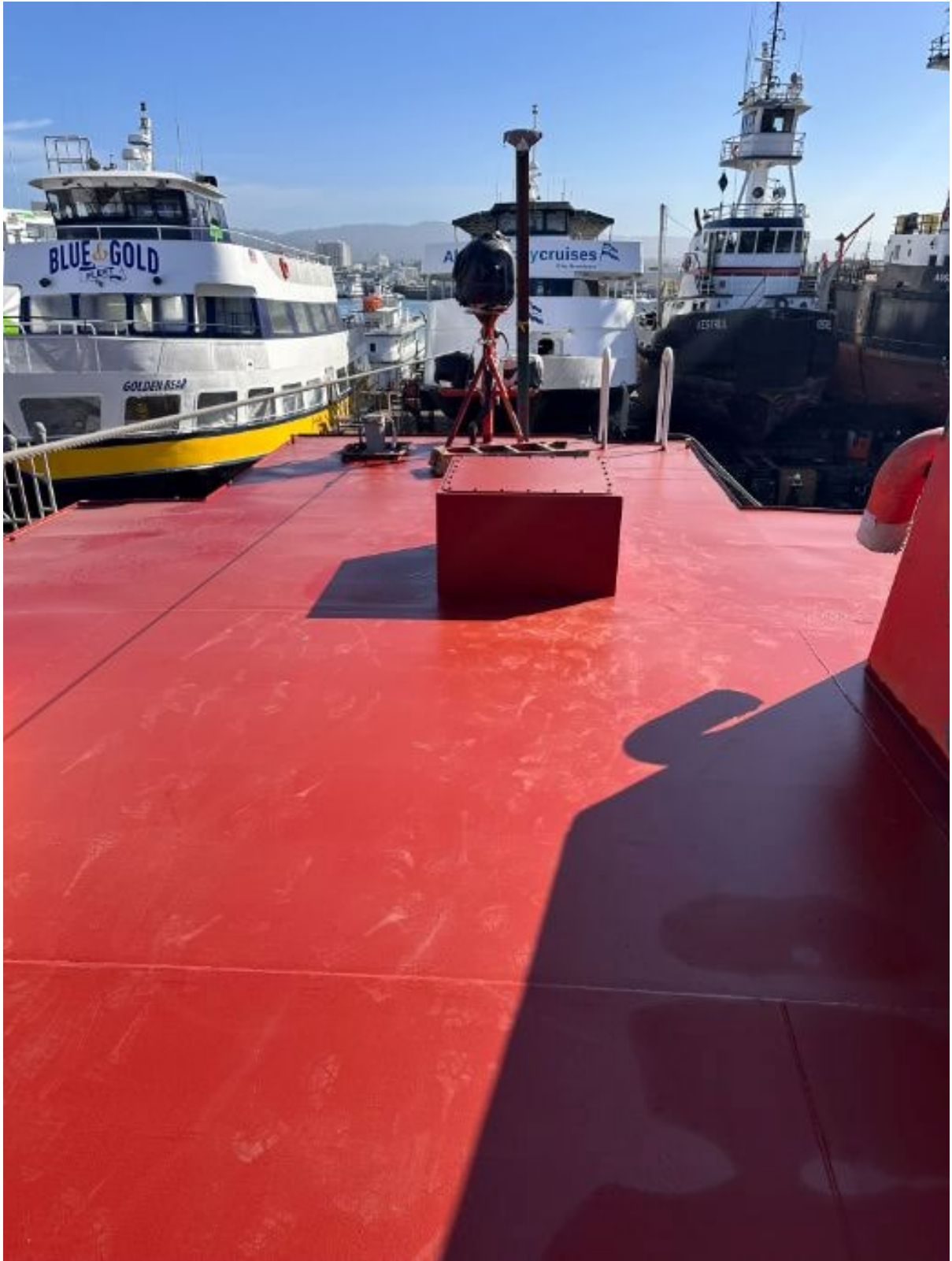
Overhead Deck After Repairs
