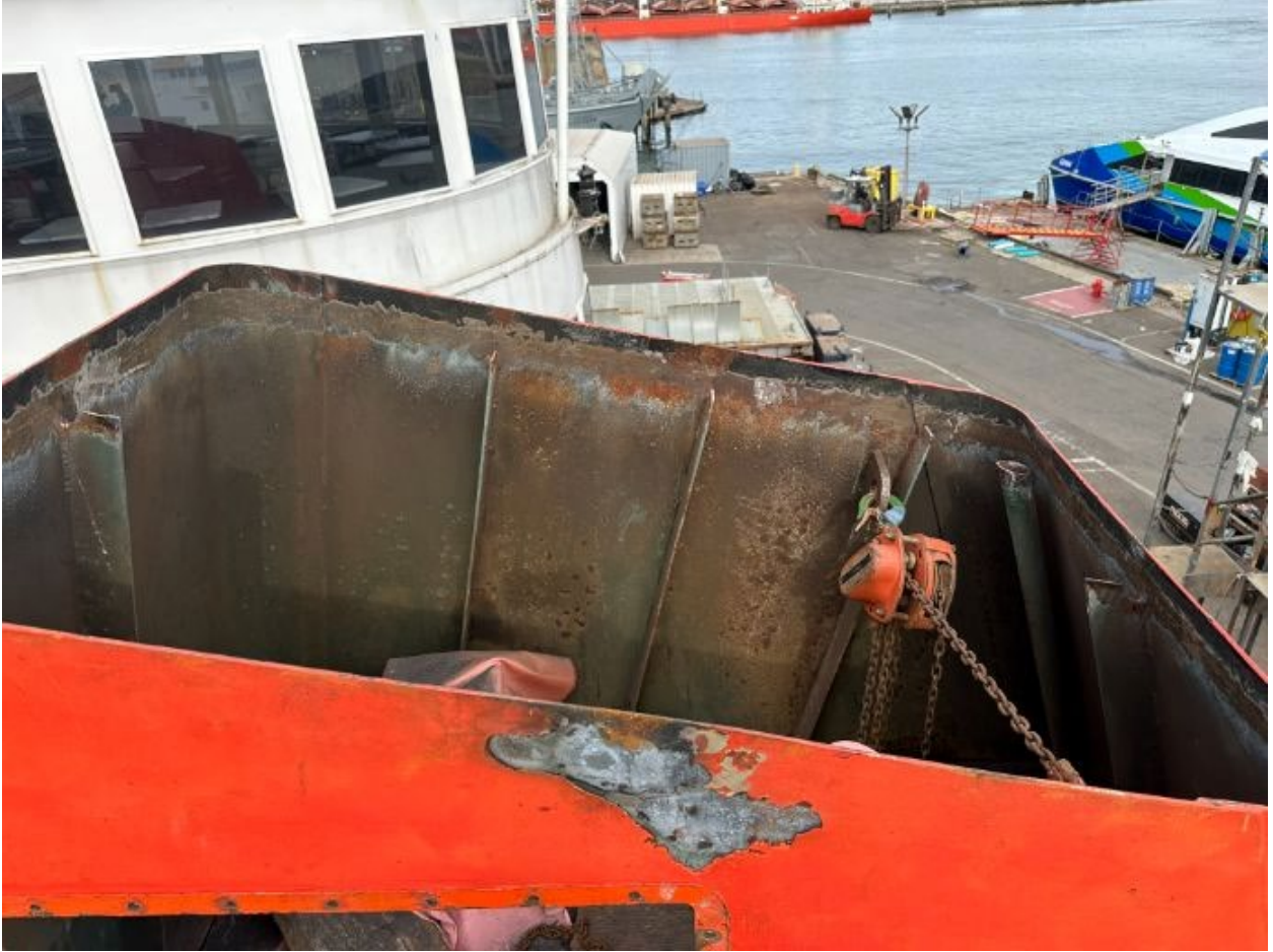
Stbd Exhaust Stack - Area of Repair
