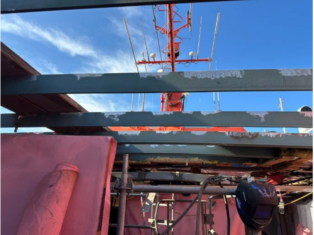
Area of Overhead Deck Repair
