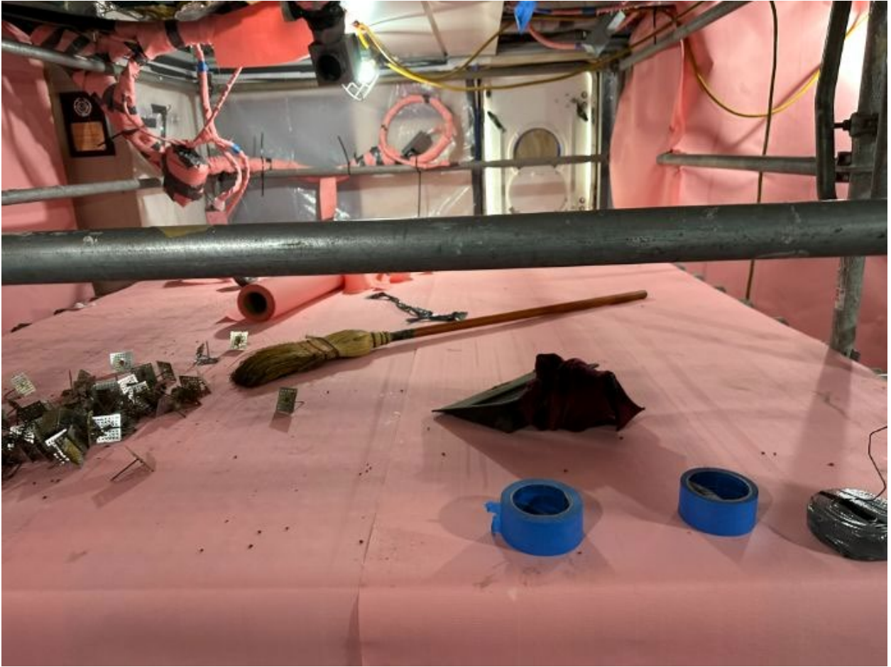
Lounge - During Repair
